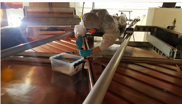
Taneli Kalvas installing the central region of the K130 cyclotron.
