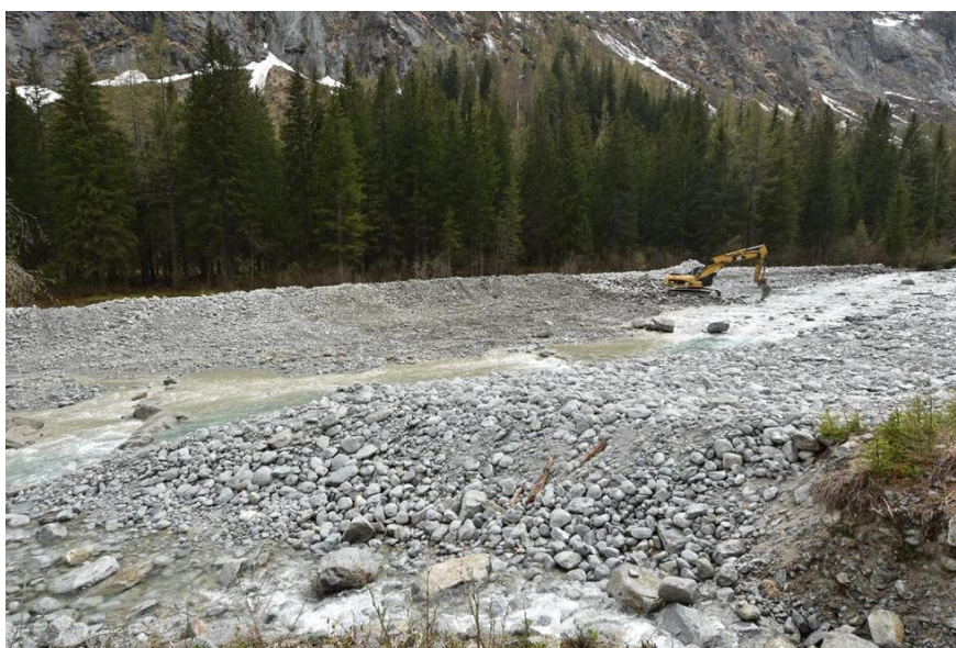
Figure 15: Heavy damage of riverbed and banks in Rio Bedù di Villa-Val San Valentino
